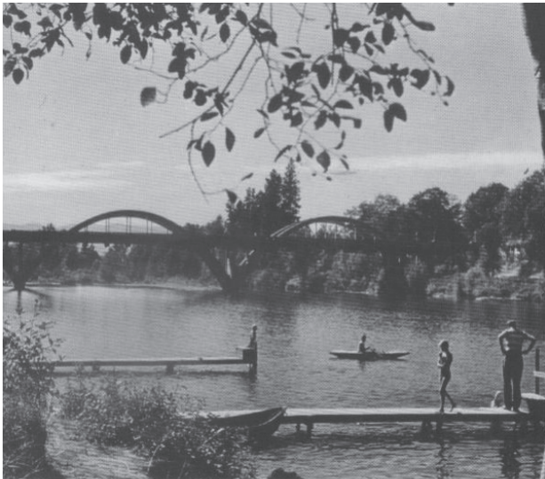
Caveman Bridge in Grants Pass before Seventh Street Bridge was built.
